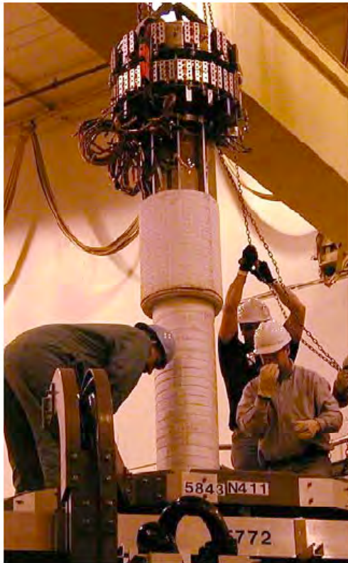
Fig. 7.3 Center-stack being installed
