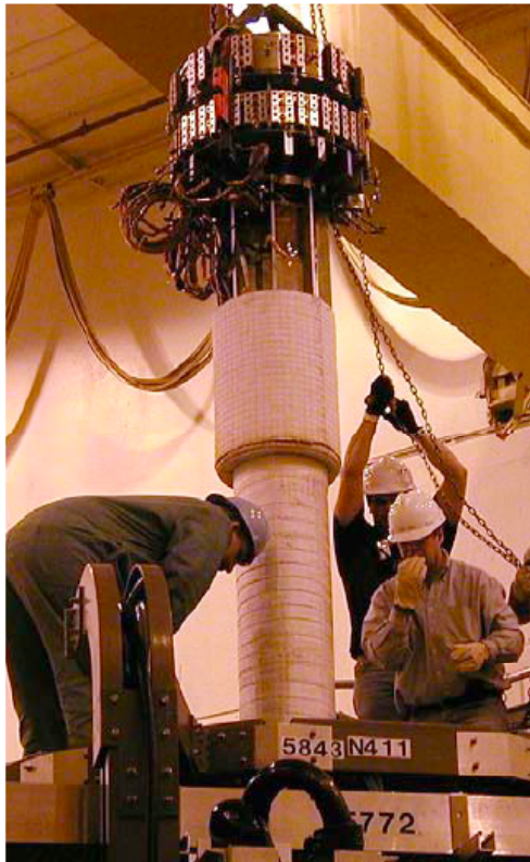
Fig. 7.3 Center-stack being installed
