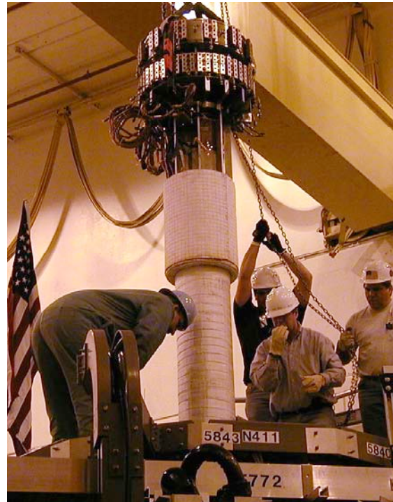
NSTX center-stack magnets lifted out of device for maintenance
