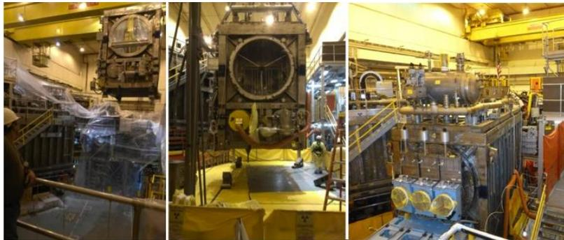
*Fig. 10.15. Relocation of the 2<sup>nd</sup> NBI beam line box. (a) The beam box lifted over the NSTX-U Test Cell. (b) The beam box being lowered into the final position in the NSTX-U Test Cell. (c) The beam box being assembled.*
