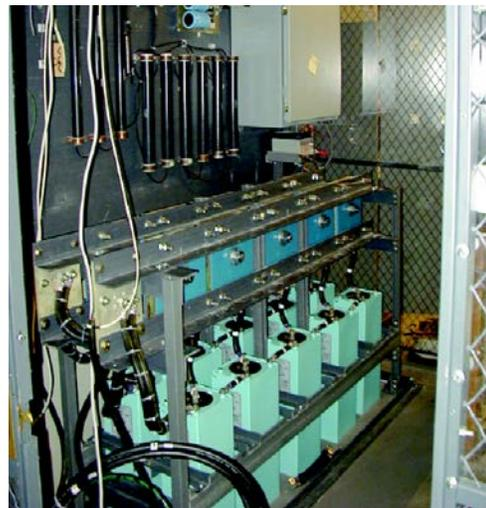
Figure 2.2.3.2.3-4: The NSTX CHI capacitor bank system is well suited to powering the EPI injector for NSTX-U.
