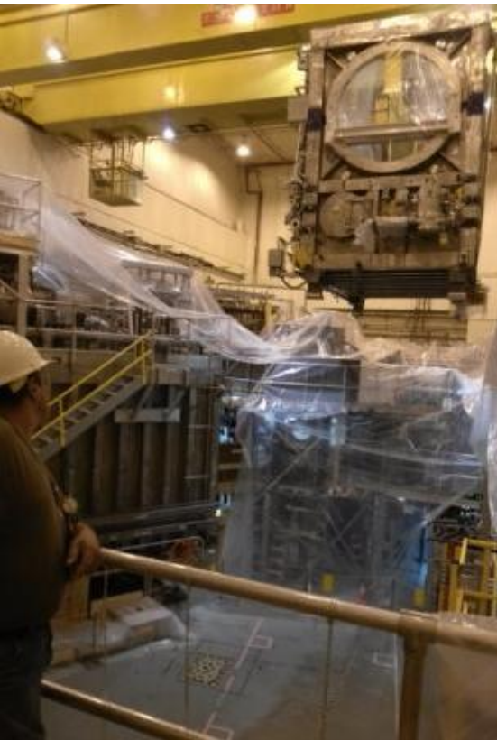
Beam Box being lifted over NSTX
