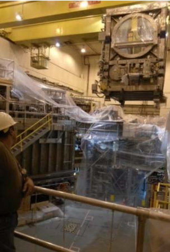
Beam Box being lifted over NSTX-U
