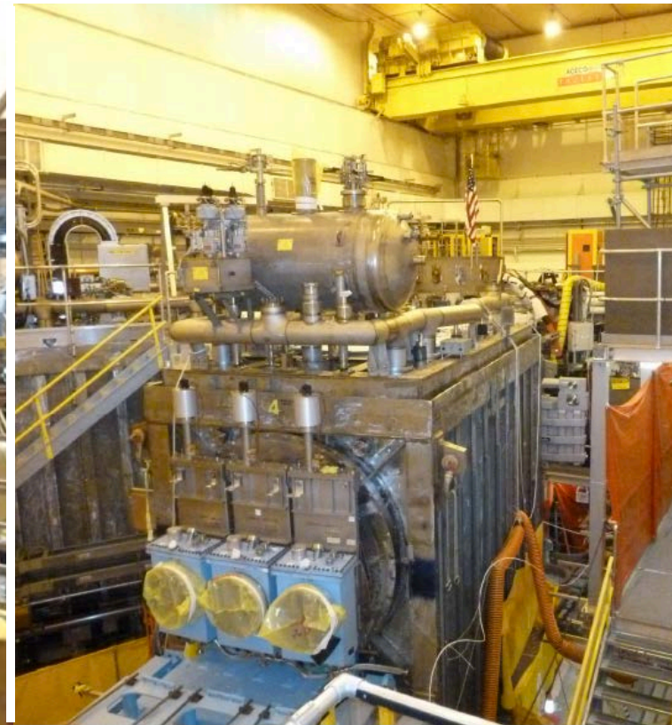
Beam Box being populated with components
