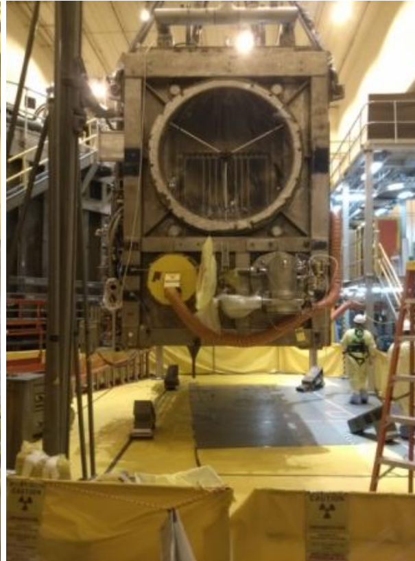
Beam Box placed in its final location & aligned
