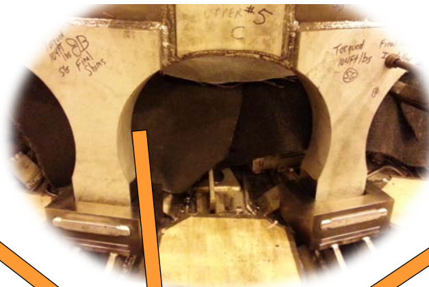
Upper Umbrella Arch Reinforcements
