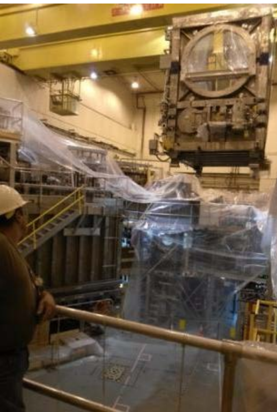
Beam Box being lifted over NSTX
