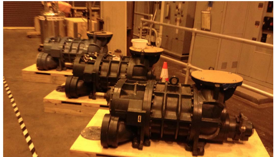
Three Helium refrigerator compressors were removed and prepared for shipment to go out for full rebuilds.
