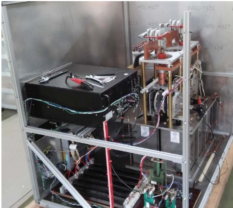
Figure IS-SFPS-3: The Univ. of Washington designed and built QUEST CHI capacitor bank (30 mF, 2kV) undergoing commissioning tests at the QUEST facility in Kyushu University during March 2016.
