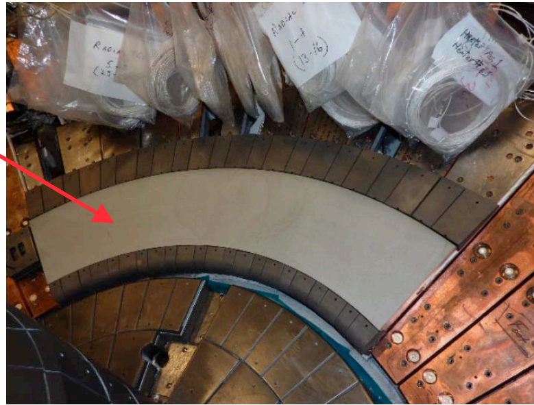
1st LLD Plate Installed in NSTX
