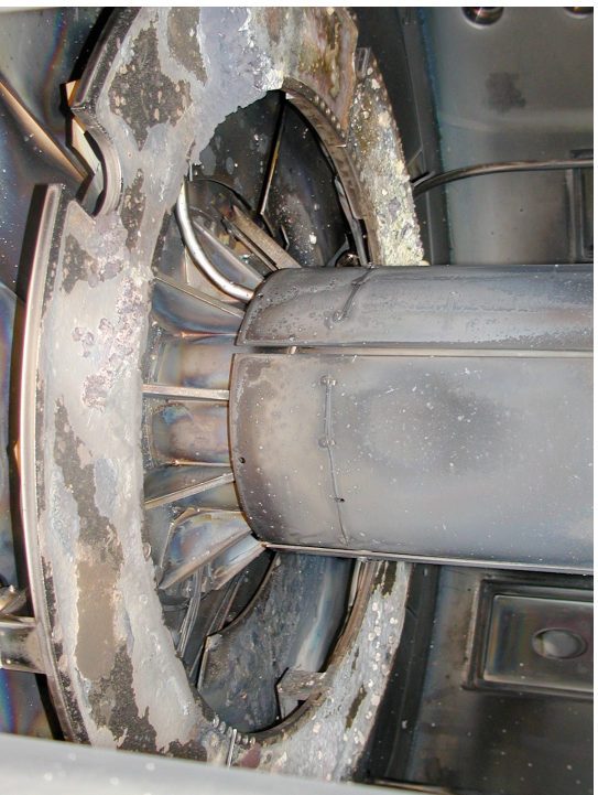
After vent but before cleaning
