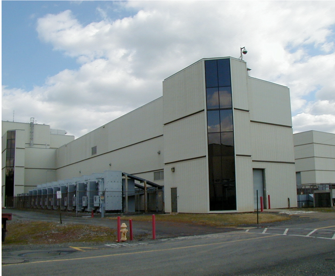
D-Site Power Conversion and MG Buildings
