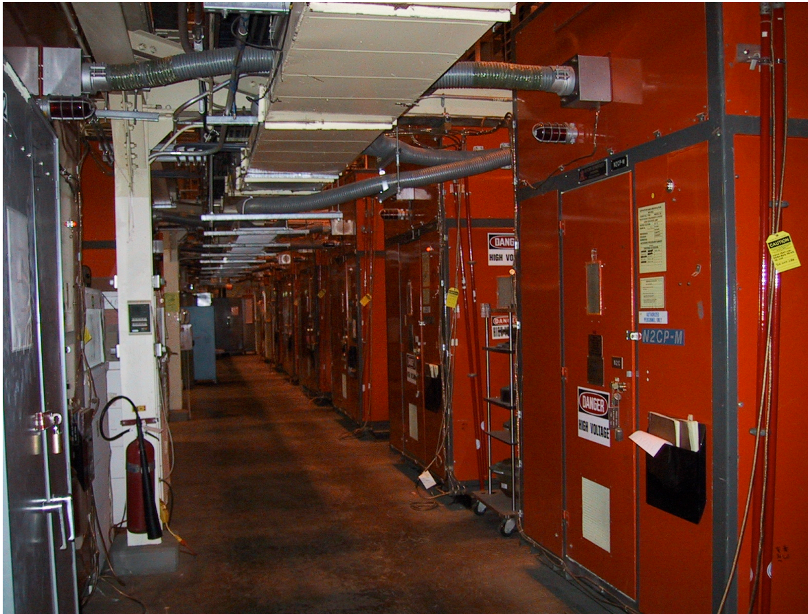
Neutral Beam Modulator Regulators for the 7MW Neutral Beam Injection (NBI) Heating System
