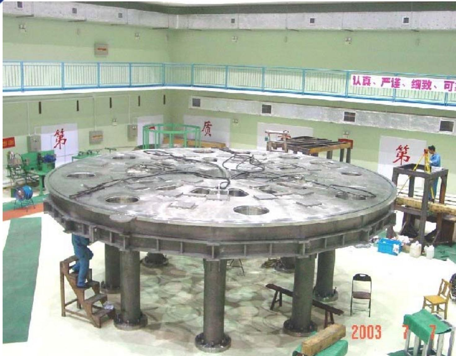
**Bottom cryostat installed on the support**
