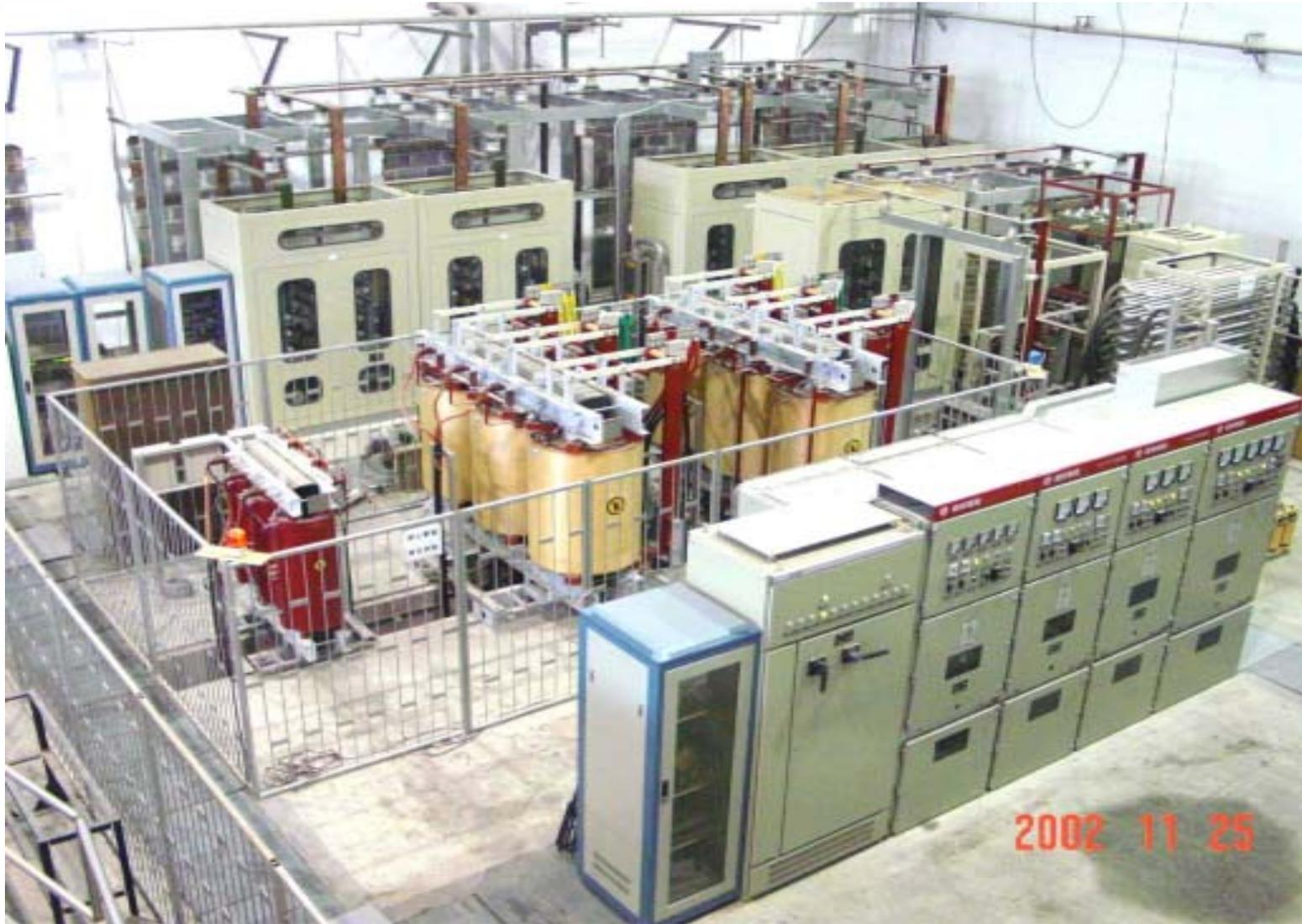
**One set of PF power supply of EAST is under testing**
