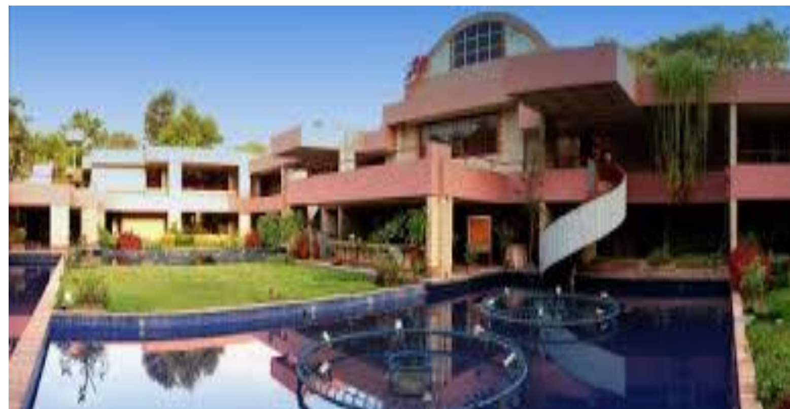
Main Building, IPR Gandhinagar
