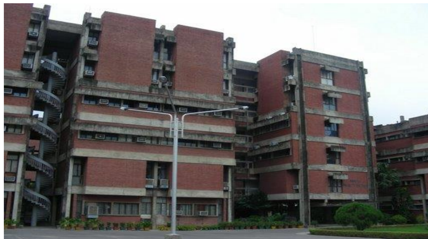
Faculty Building, IIT Kanpur
