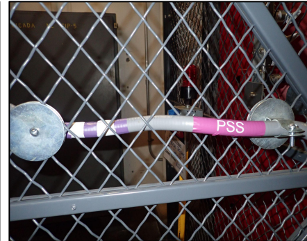
CONDUIT LABELING IN THE FIELD
