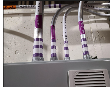
CONDUIT LABELING IN THE FIELD
