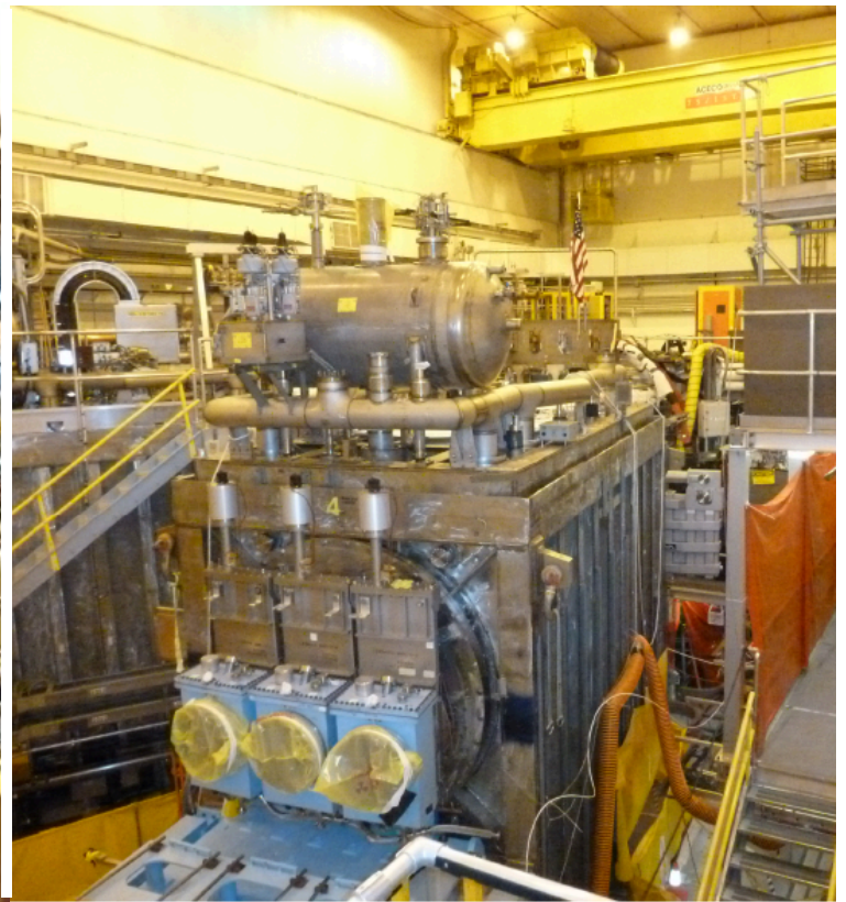
Beam Box being populated with components
