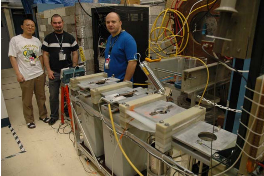
(1 mF, 10 kV capacitor bank)
