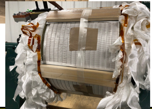
Everson-Tesla completed last layer and have brazed outer flag
