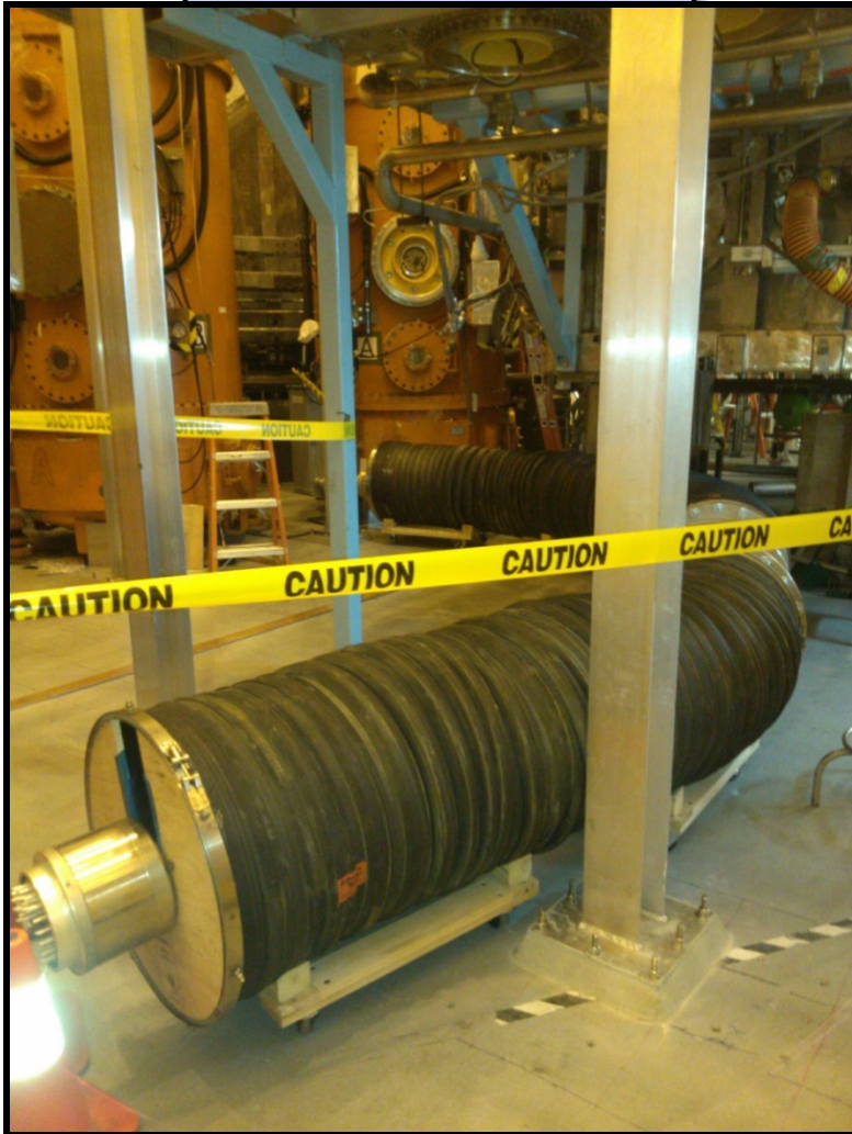
Transmission line installation
