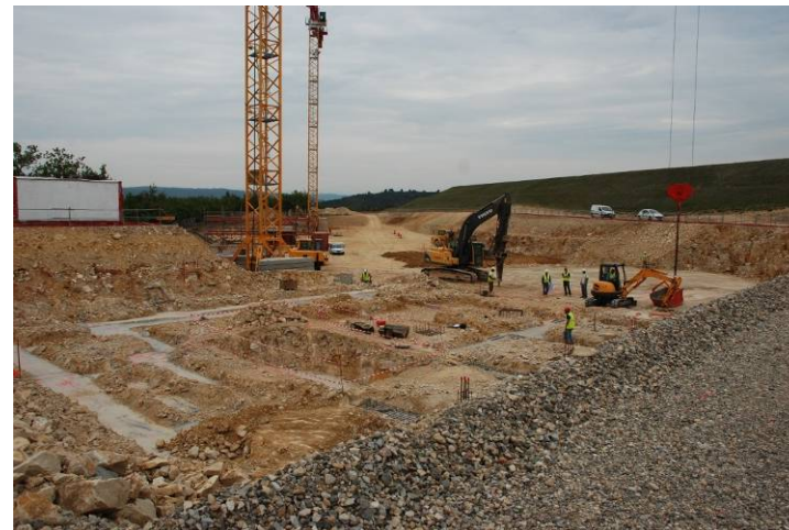
Excavation of the Tokamak Building
