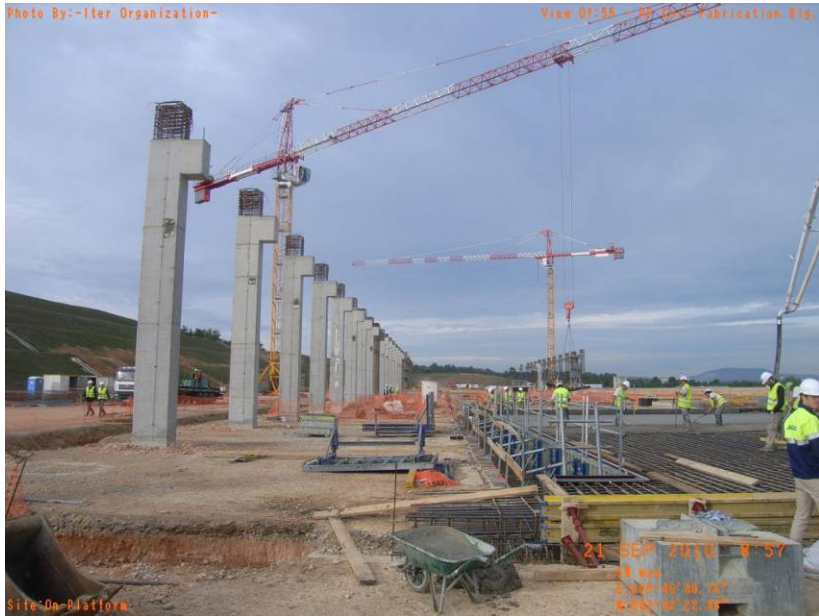
The concrete foundation for the Poloidal Field Coil Winding Facility is being put in place
