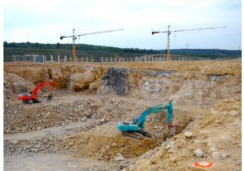
Excavation of the Tokamak Building
