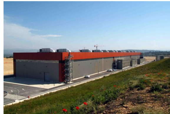
Poloidal field coil winding building
