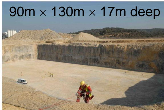
Tokamak seismic pit and foundation
