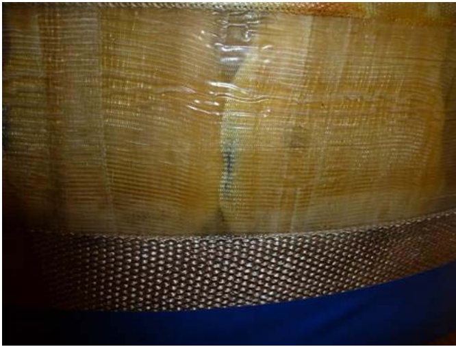
Fig. 5. PF1A-U ground wrap delamination.
