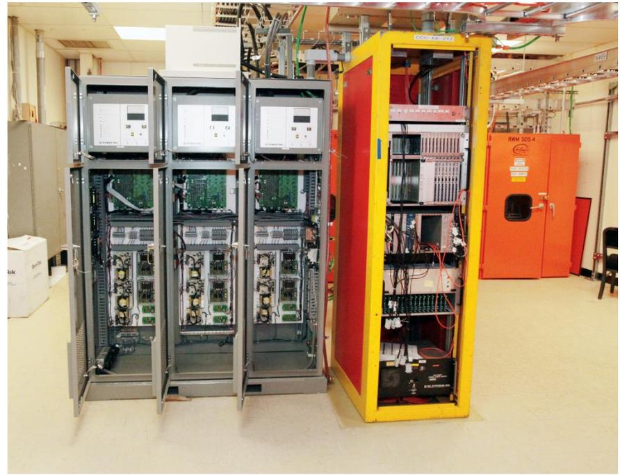
2nd 3-channel Switching Power Amplifier (SPA) commissioned in July 2011 powers independent currents in six EFC/RWM coils for simultaneous control of  $n = 1, 2, 3$  field harmonics
