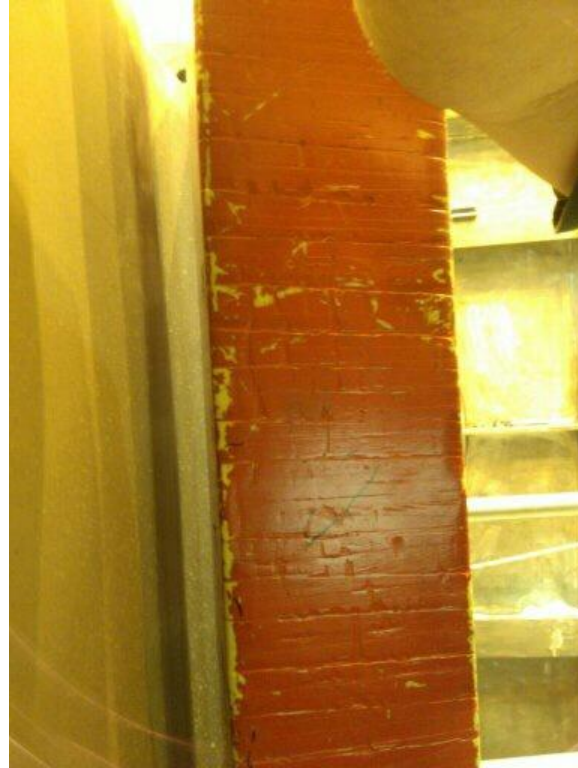
Maintained \frac{3}{4} inch clearance to Port Extension for OL deflection per spec
