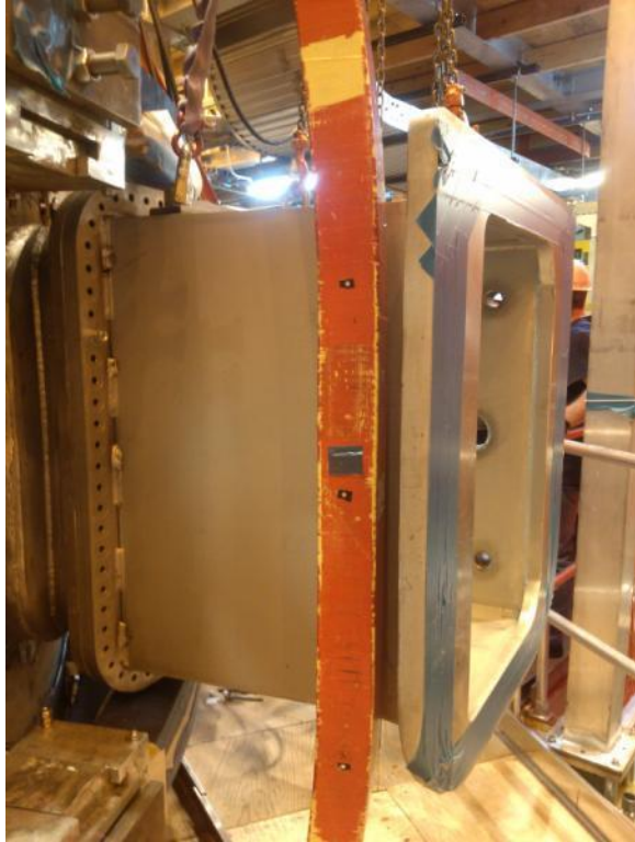
TF outer leg clearances maintained
