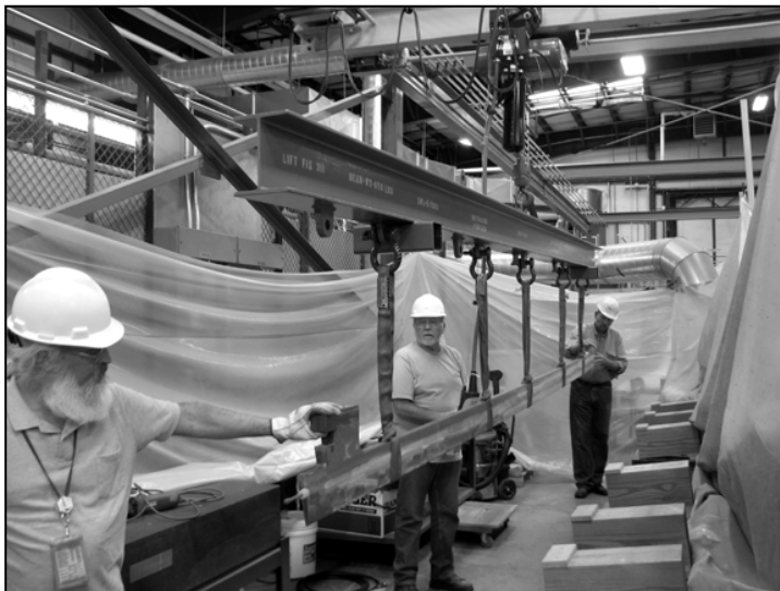
Fig. 5 Finished TF Conductor Being Removed from Grinding Area
