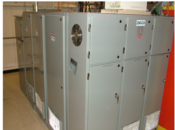
Figure 6 View of the front of SPA-2
