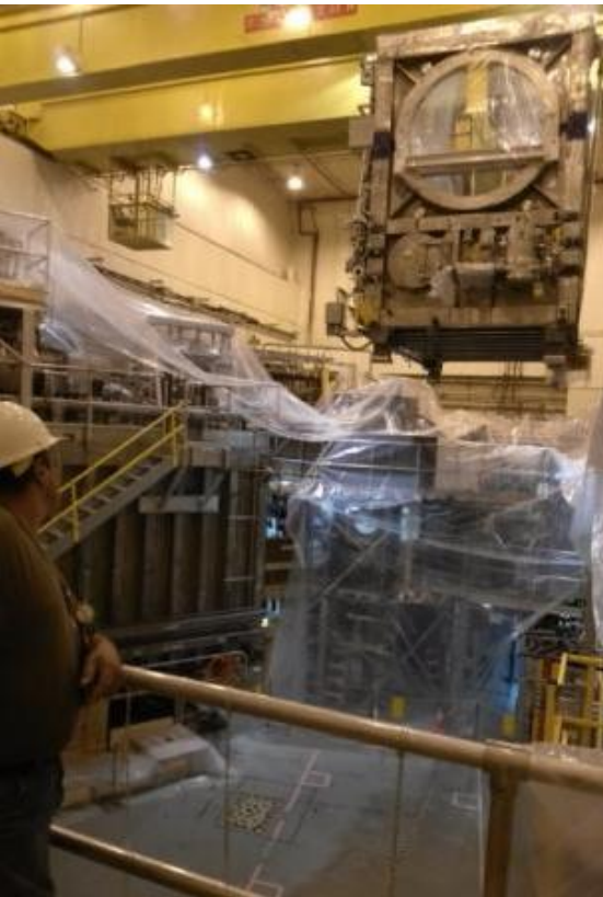
Beam Box being lifted over NSTX
