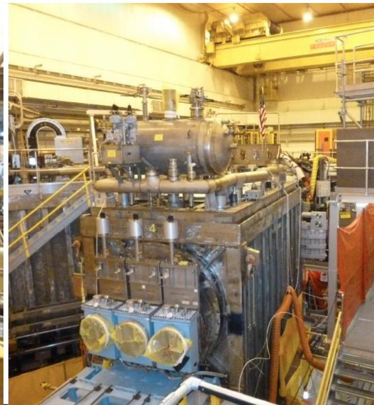
Beam Box being populated with components
