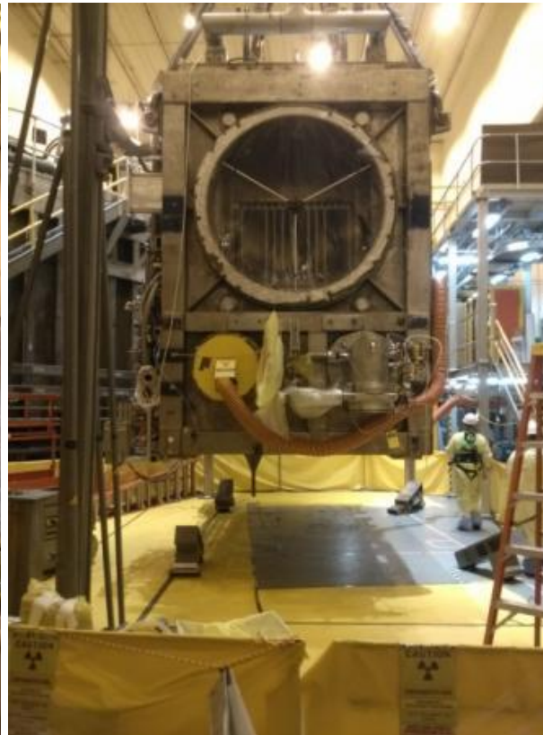
Beam Box placed in its final location and aligned
