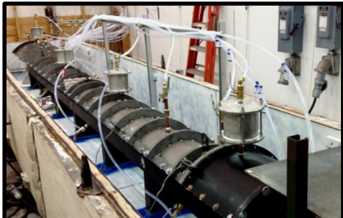
Assembled TF mold ready for Vacuum Pressure Impregnation (VPI) w/ CTD-425
