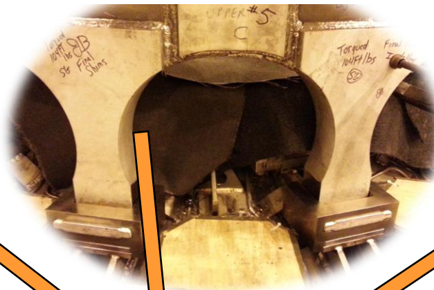
Upper Umbrella Arch Reinforcements
