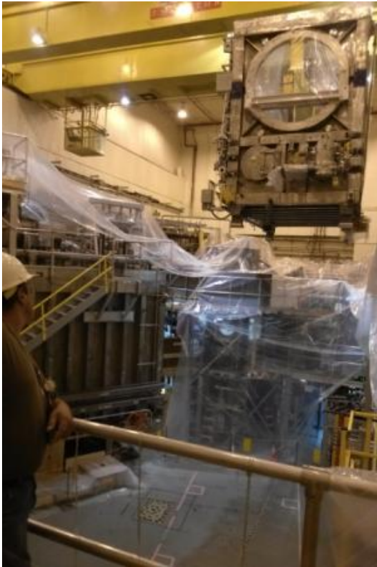
Beam Box being lifted over NSTX
