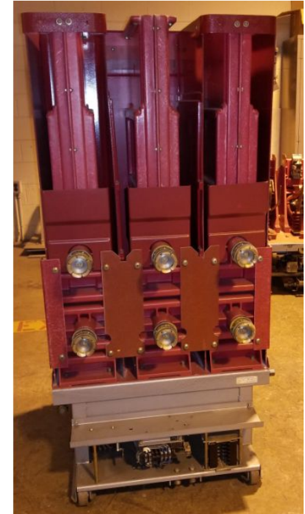
SV Lineup breaker (500MVA) withdrawn from cubicle
