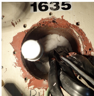
Installation of Neutron Putty
