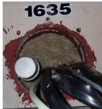
Installation of Rockwool
