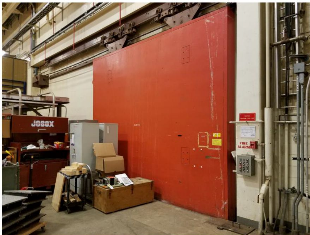
Figure 2-8: Photograph of the neutral beam power conversion mobile shield door, from the power conversion building. The south high bay is on the other side of the door.
