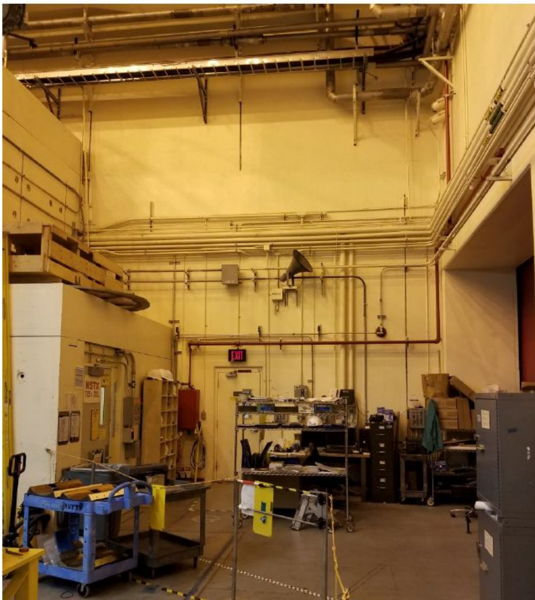
Figure 2-7: Photographs of NSTX-U South High Bay, looking toward the door to the east gallery. The neutral beam power conversion building mobile shield door is on the right of the figure. The NSTX-U device is on the left on the other side of the shield wall. The personnel door beneath the exit sign is a primary source of neutron leakage from the test cell.
