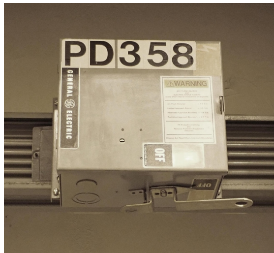
Figure 1. Bus Duct Disconnect Switch
