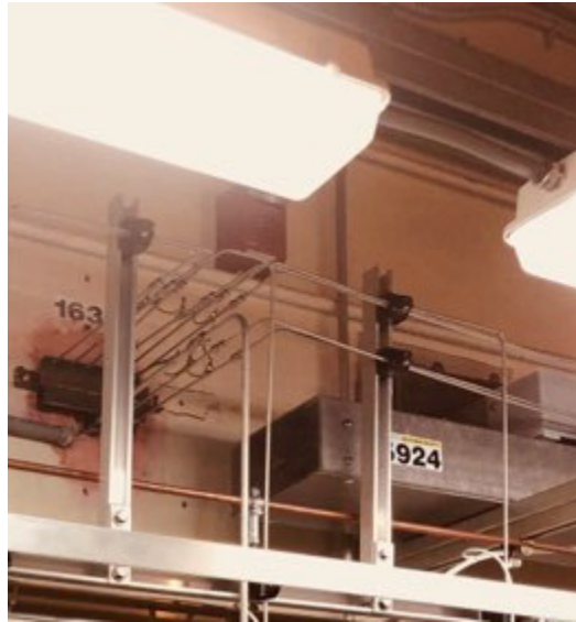
Figure 4. Gas tube penetrations
