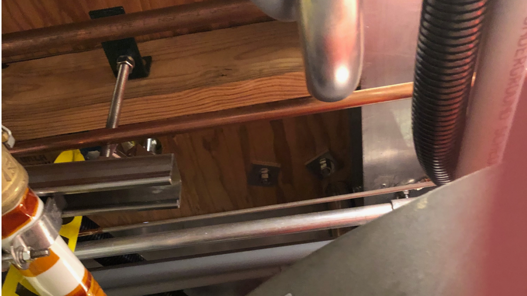
Figure 3. Water Lines feeding manifolds supported from platform
