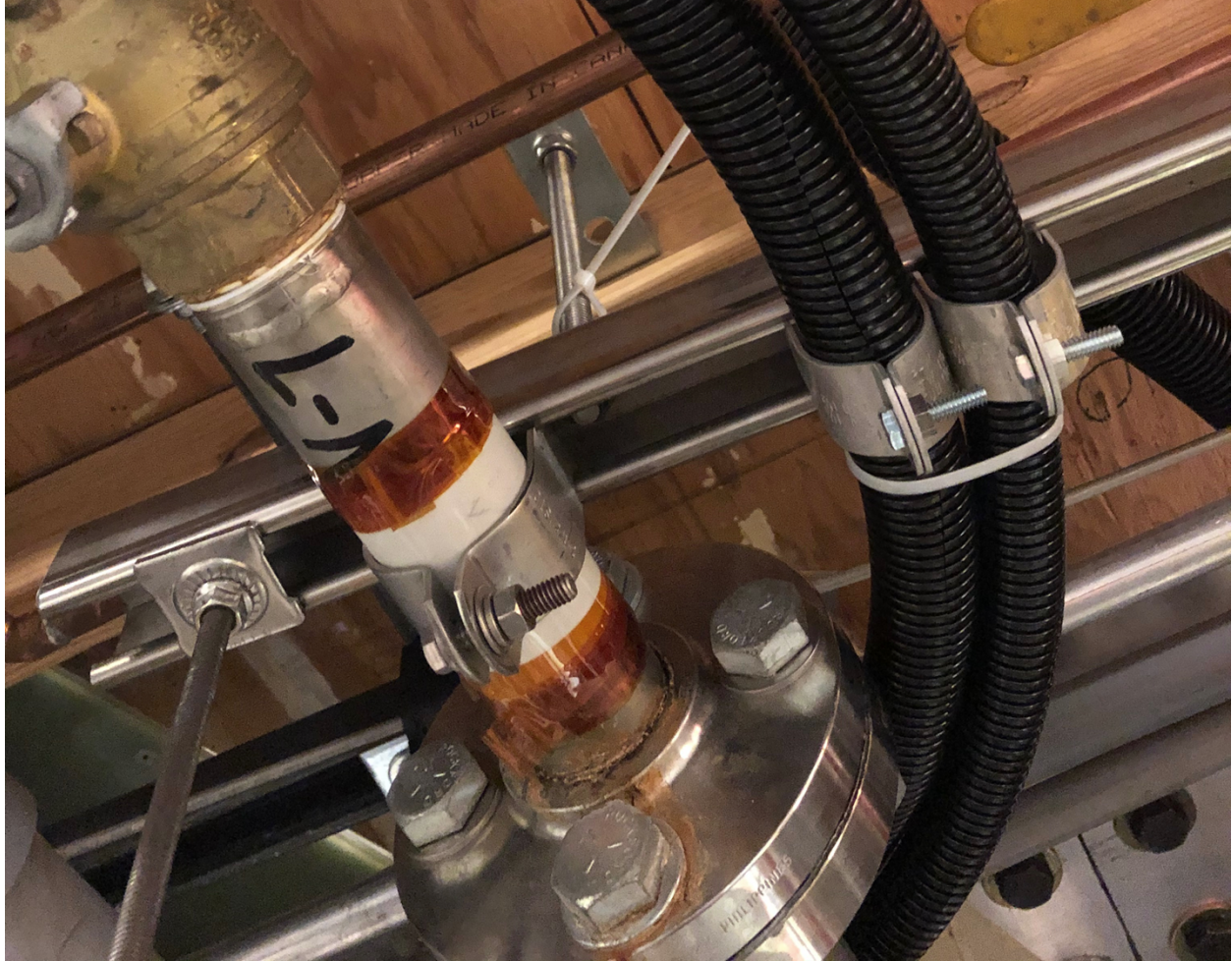
Figure 1. Pipe hanger supported from platform
