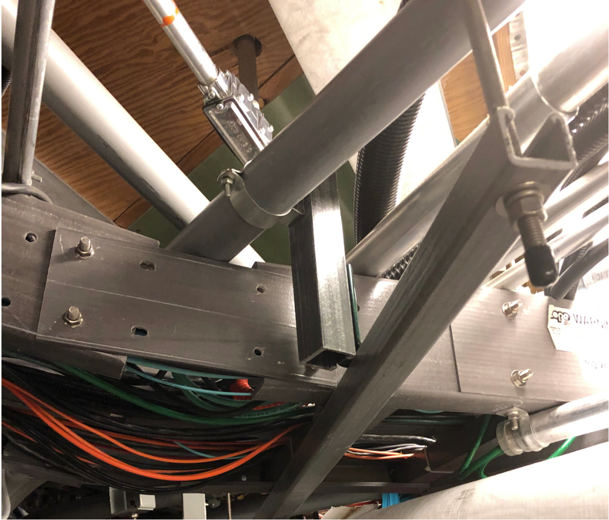
Figure 5. Cable trays contain PLC wiring
