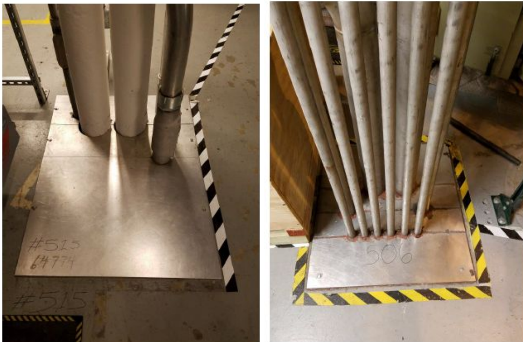
Figure 2-14: Photograph of the neutral beam water pipes as they pass through the penetration in the test cell floor. The left image is of penetration 515, while the right image is of penetration 506.
