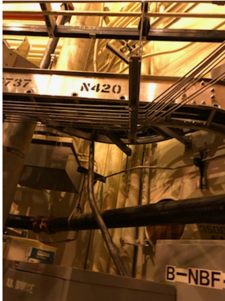
Figure 3. Gas lines attached to cable trays
