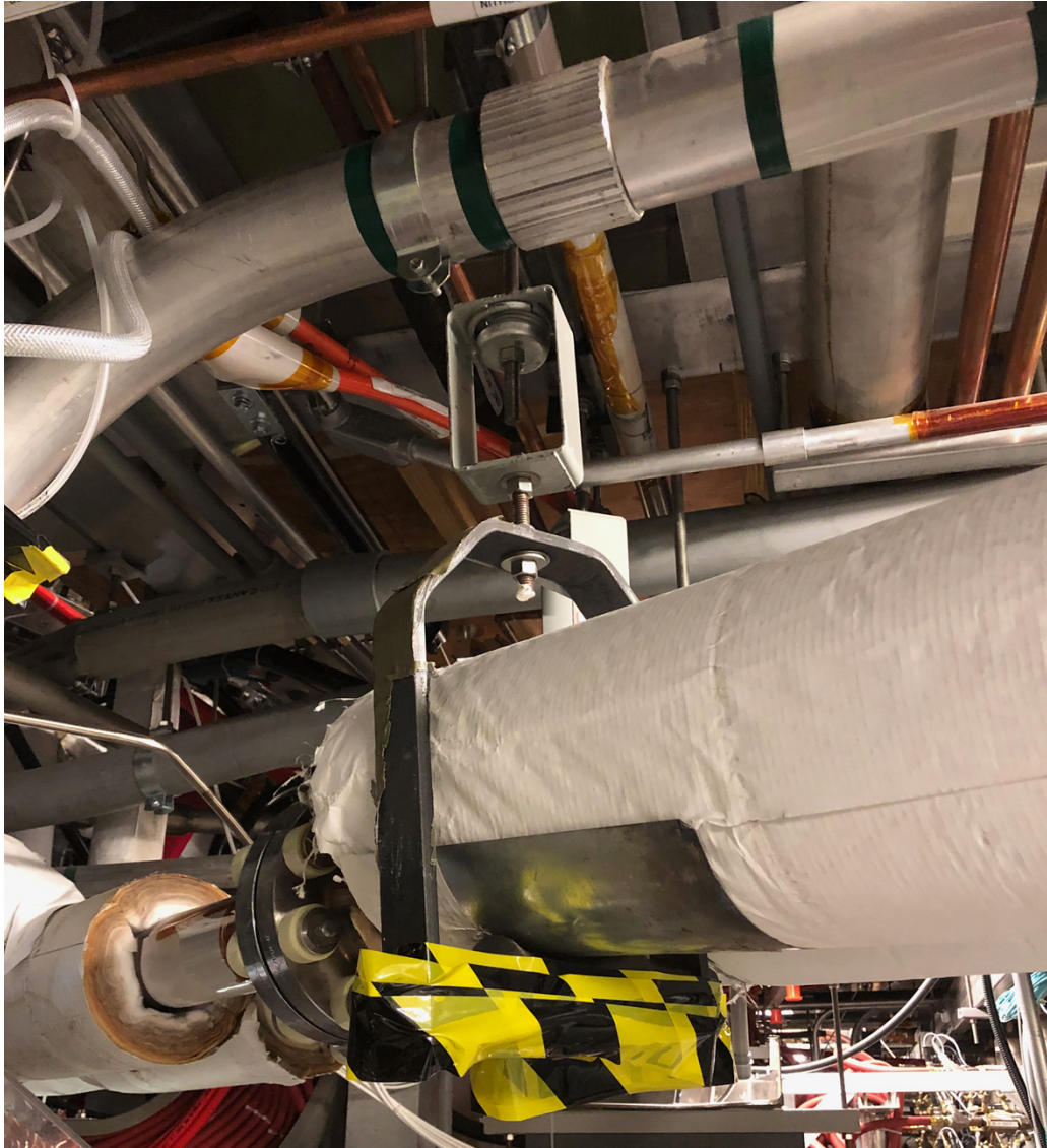
Figure 4. Helium lines feeding the manifold supported from platform
