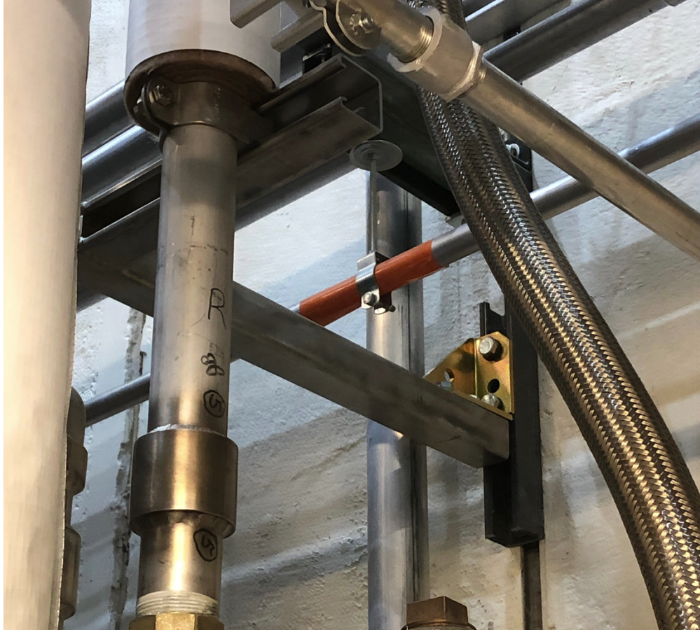
Figure 2. Pipes supported by the wall
