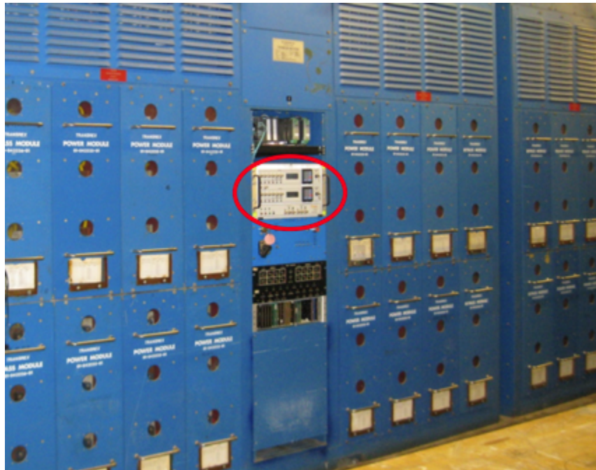
Figure 6. Notional Rectifier with Firing Angle Receiver and Computer
