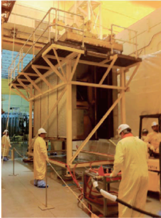
2 nd NBI lid being prepared for lift in the NSTX-U Test Cell South High-Bay Area
